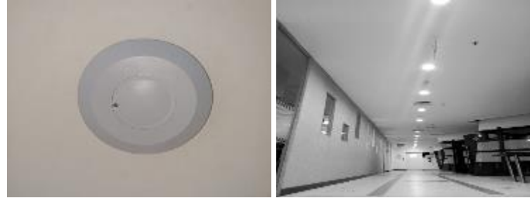
Installation of Motion Sensor for passage and common area lighting system
