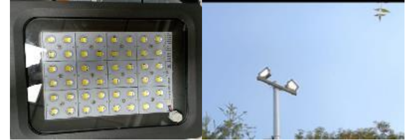
Replacement of 400 W X 12 no's Metal Halide Type (Flood Light) with LED light 250W
