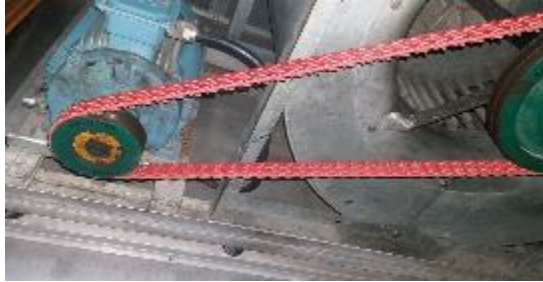
Replacement of conventional AHUs with EC Fans
